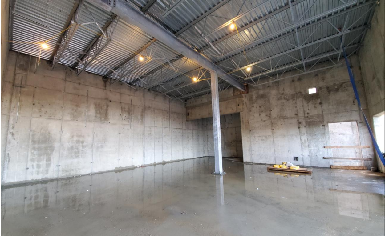
Water Treatment Plant Workshop and Storage Room
