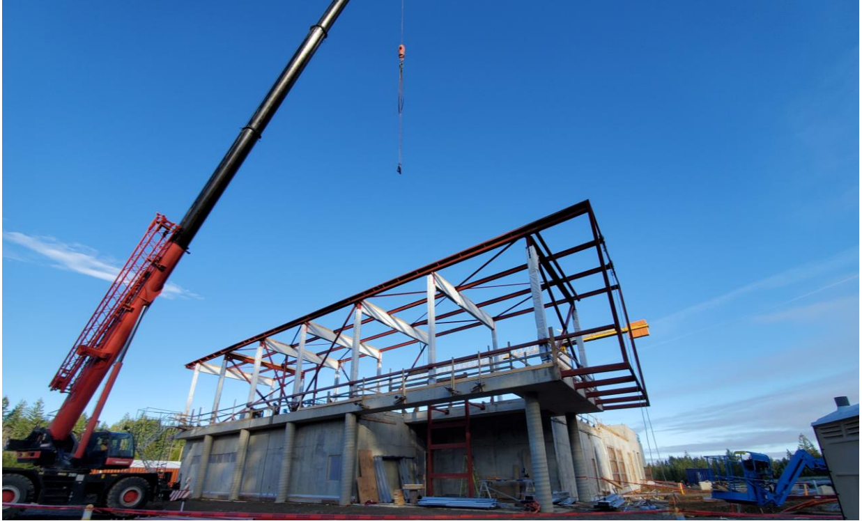
Water Treatment Plant lobby steel and glue-lam beams being erected
