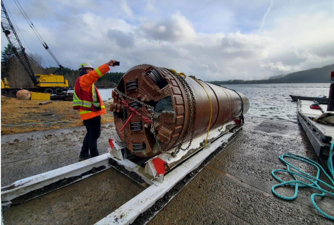
Tunneling machine, sitting in the cradle, retrieved from the lake after completion
