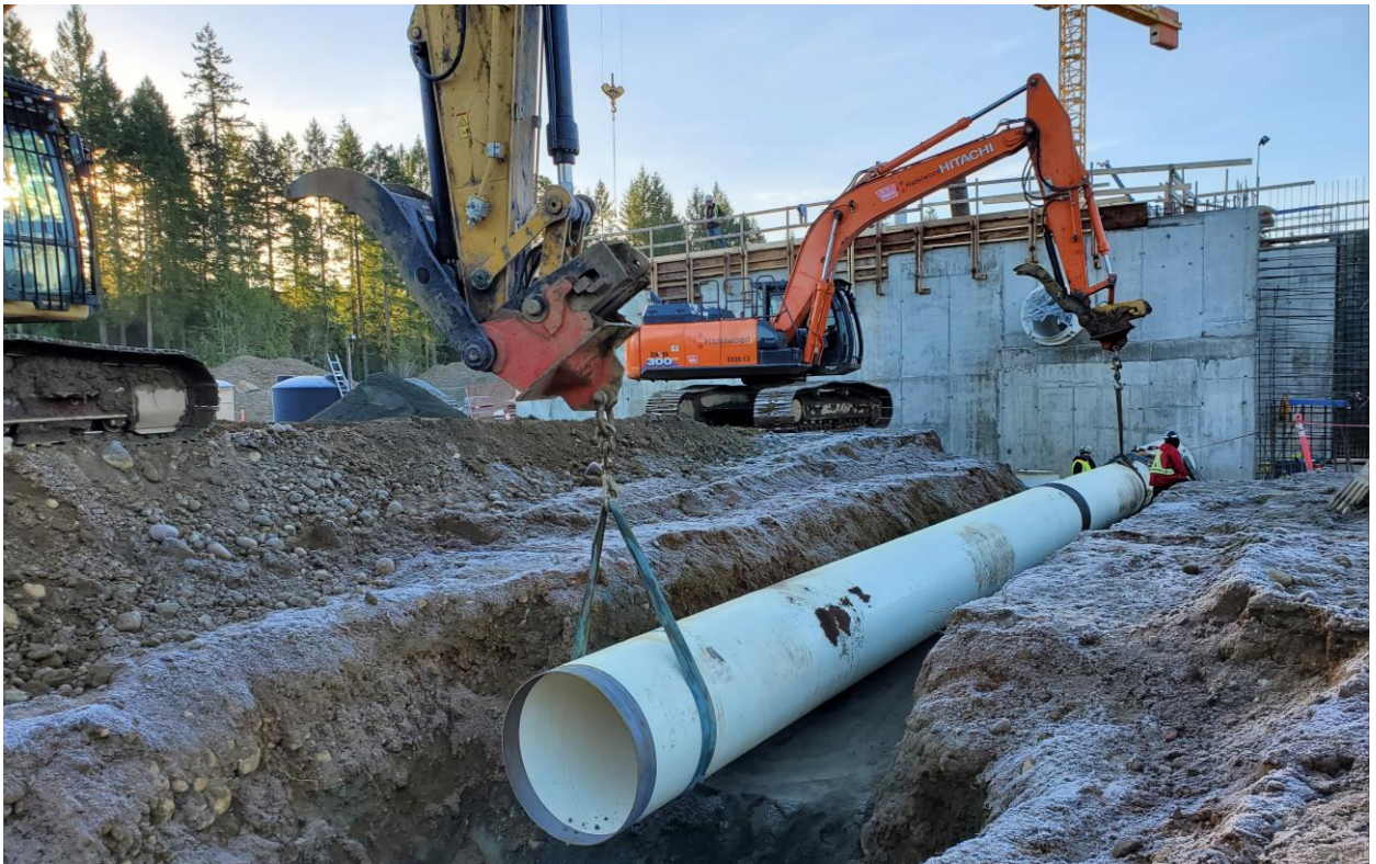
Treated Water Transmission Main being connected to Clearwell at WTP
